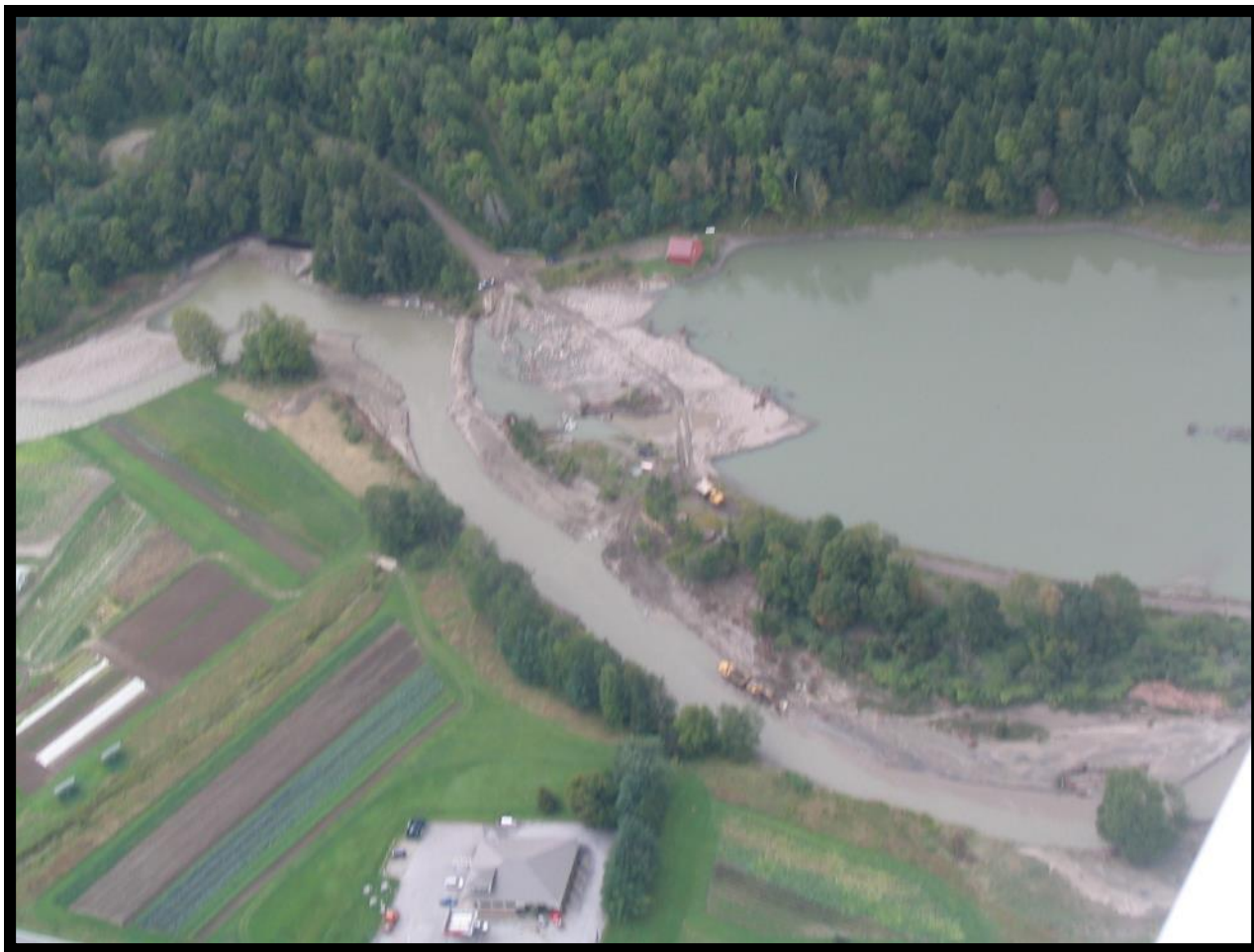
Figure 1 Sugarbush Snowmaking Pond. River avulsion damage after Tropical Storm Irene.
